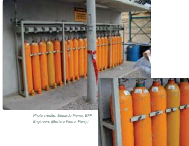
Restraint for Gas Cylinder Against Wall Image credit: FEMA 74
