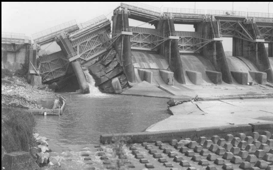
The 1999 Chi-Chi earthquake, Shih-Kang Dam
