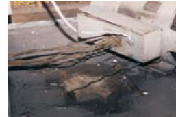
Broken electrical connections resulted from large displacement of an improperly anchored lift generator (left); view of one of four generators moved from anchorage, 1994 Northridge, California earthquake (right).
