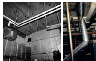
Photo credit: Mason Industries Fallen ductwork (left) and (right); duct crushed by swinging pipes (center) 1994 Northridge, California earthquake.
