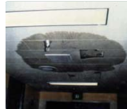
Photo credit: Degenkolb Engineers, FEMA 74
