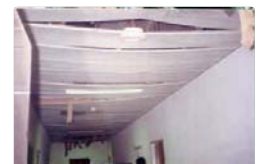
Photo credit: EERI 2003 Bam, Iran Earthquake Reconnaissance Report Damage to an operation theatre ceiling at Kona Community Hospital, 2006 Hawaii earthquake (left); buckled panels in a hospital corridor suspended metal panel ceiling, 2003 Bam, Iran earthquake (right).
