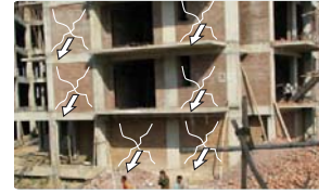
Photo credit: Melvyn Green, Melvyn Green and Associates
