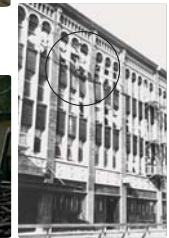
Photo credits: NISEE (Karl Steinbrugge and Harold M. Engle)
