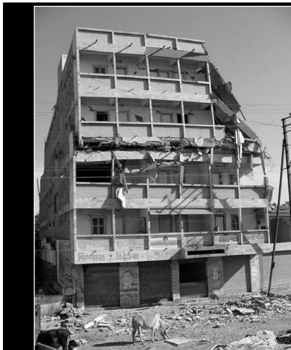
Intermediate Story Collapse in a 6-story Building in Bhuj
