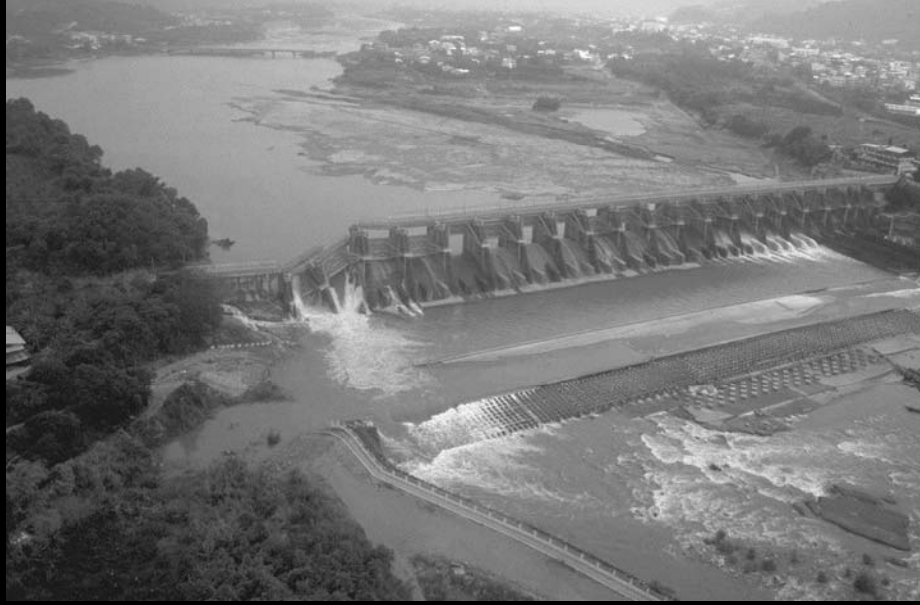
The 1999 Chi-Chi earthquake, Shih-Kang Dam
