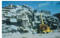
Collapsed Hospital Juarez (left) and Hospital General (right) Mexico.
