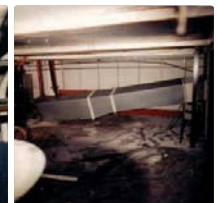
Photo credit: Mason Industries Fallen ductwork (left) and (right); duct crushed by swinging pipes (center) 1994 Northridge, California earthquake.
